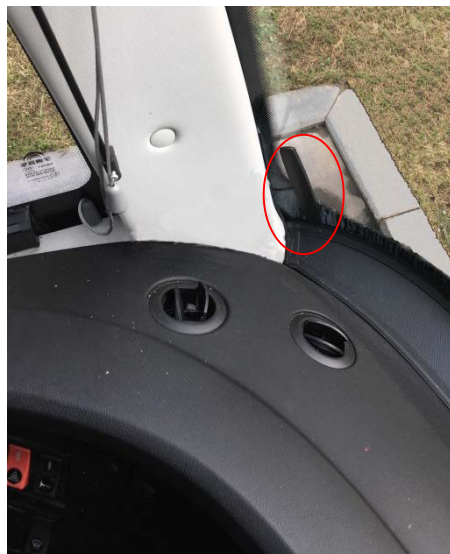
Figure 2-24 Inside installation of Mobile Network Antenna
